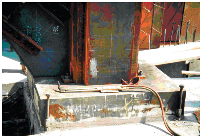
Figure 2.2. Base plate with adjusting screws.
